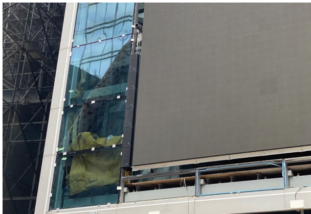
SIX RENKUS-HEINZ ICLIVE X DIGITALLY STEERABLE ARRAY MODULES COVERING THE NORTH SIDE OF MAPLE LEAF SQUARE
